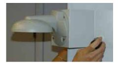
• Attach the assembly to a wall corner with dry wall anchors and machine screws.
