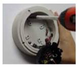
2 Mount the surface mount with the included machine screws.
